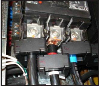
Figure 7. CT Connection Points (300 A CT Shown)
